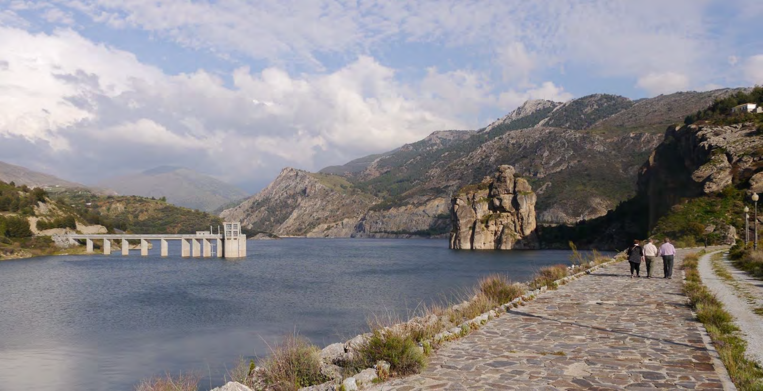
Hydropower plant Canales, Andalucia, Spain (Source: Dirk Oudes)
