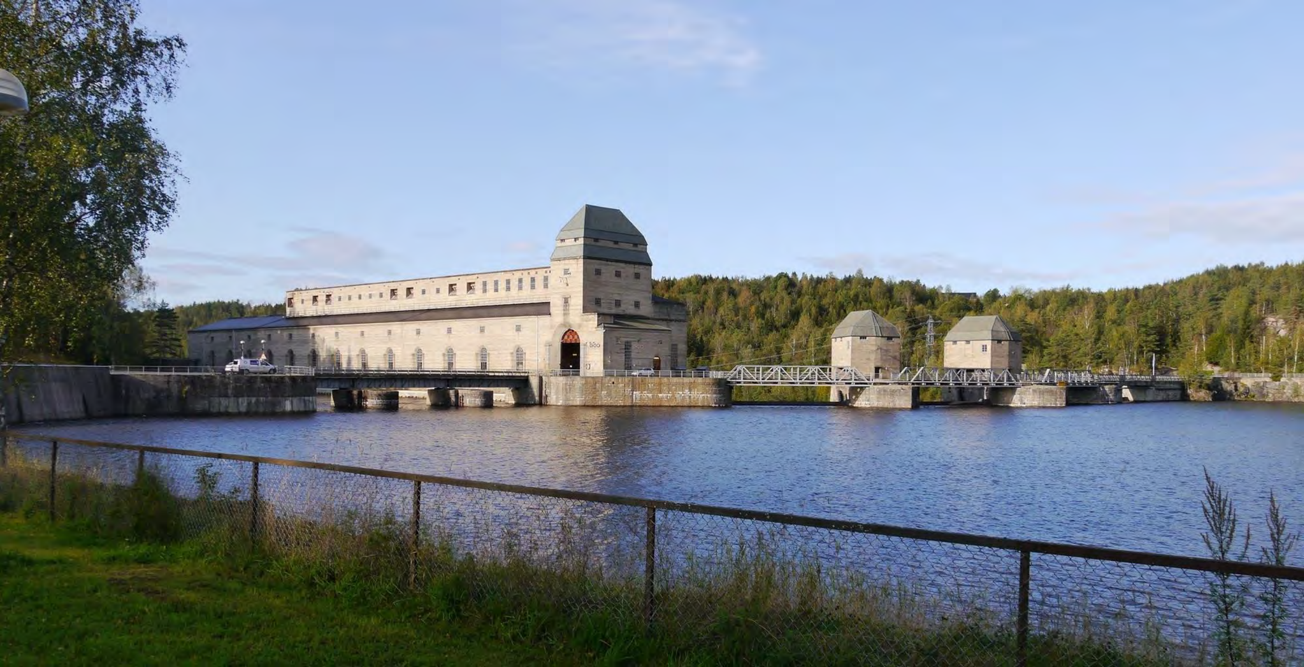
Hydro power plant Solbergfoss built in 1924, Norway (source: Dirk Oudes)
